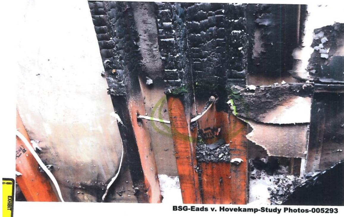
Mr. Gary Woodall will testify at trial that he has examined all of the evidence and believes the most likely cause of the fire was the refrigerator. Mr. Woodall's opinion is consistent with the burn patterns left in the garage. Specifically, the "V" pattern which is shown by the burnt materials and which leaves the refrigerator at the bottom of the "V" pattern.
